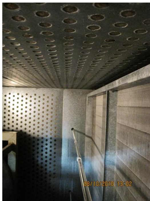
AHU T2-20 plenum with Steril-Aire very high output UVC Emitters™ installed
