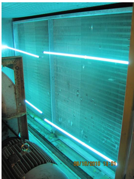
AHU T2-20 plenum with Steril-Aire very high output UVC Emitters™ installed
